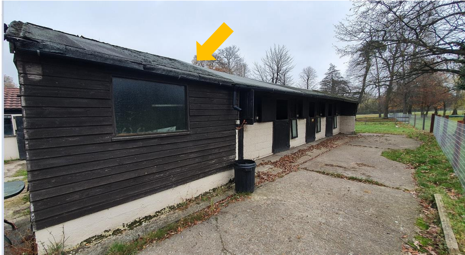
Photo 3 The existing stable (view from the north) to be demolished
