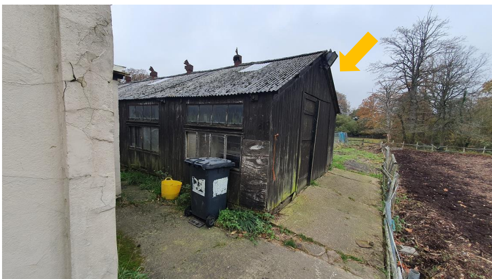
Photo 2: The existing stable (view from the south-east) to be demolished
