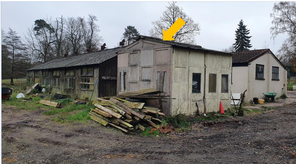
Photo 1: The existing barn (to be demolished)
